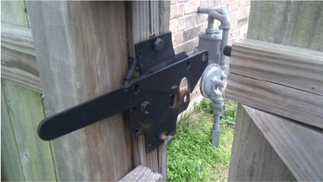
Closures common to wood privacy fences are more often self-latching as the latch closes over the arm when the gate swings shut.
